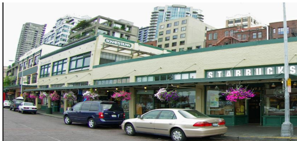
Mixed-income Housing at Pike Place Market – Soames Dunn apartments, the First, Mixed-income, Section 8 Housing Approved in the U.S.
